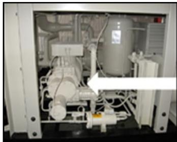
**Semi-Hermetic Rotary Helical Screw Compressors**
