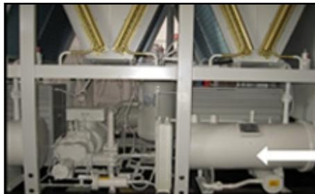
**Oversized Receivers** - used for all low ambient Chillers. Prevents cycling and operational damage of components.
