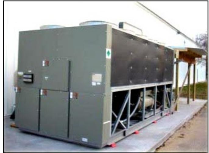
The **blü line™** chiller is air cooled and eliminates the need for an evaporative condenser which uses additional power, space, masses of water and additional inputs such as water softener, algacide, and higher maintenance costs that if forgone could create a breeding ground for pathogenic bacteria such as Legionella.
